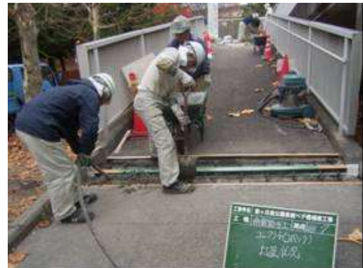
橋梁の補修工事②
