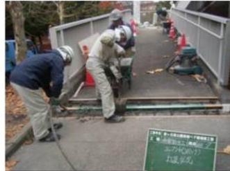
橋梁の補修工事②
